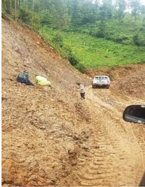
Photo taken by OAG on 4 th March 2020, showing landslides at one of the sections
